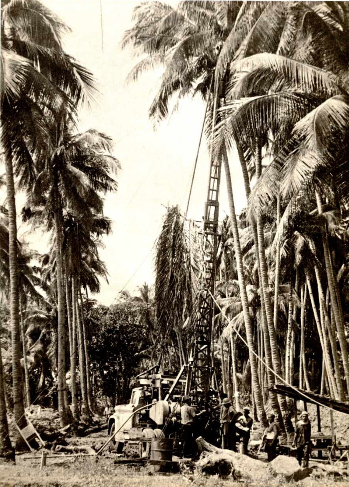
Drilling operations are underway to tap fresh water from a deepwell.
