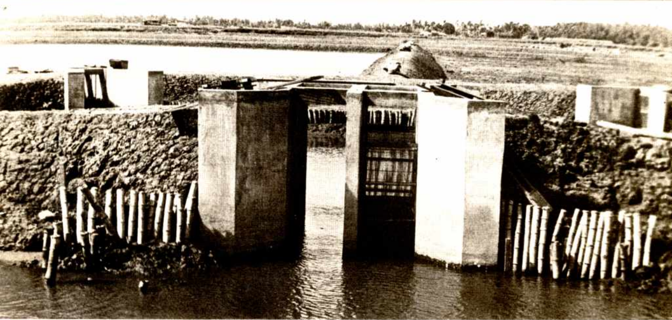
Top, A close-up of the main gate under construction; Below, One of three secondary gates with the correspond- ing tertiary gates leading to each of the ponds.
