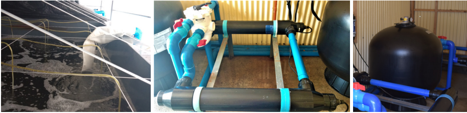
Figure 16. Seawater from the reservoir passes through various filtration and sterilization stages before reaching the larval rearing and natural food tanks.
