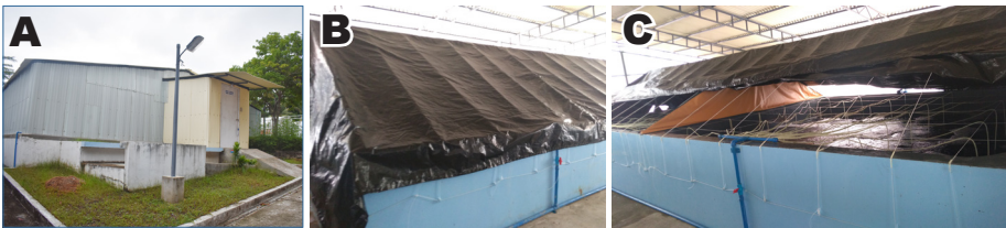
Figure 19. The larval rearing facility at SEAFDEC/AQD: A. exterior view of the facility, B. tanks completely covered with laminated black sack, and C. divisions provided between tanks.
