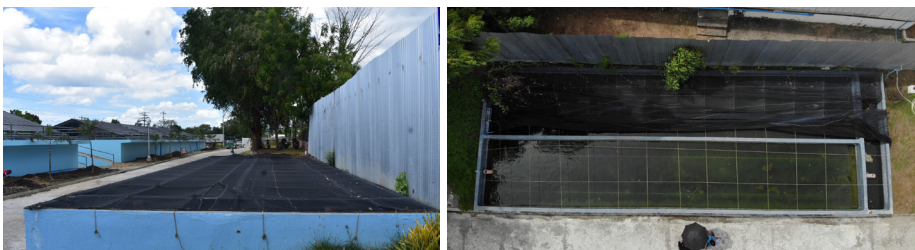
Figure 20. The wastewater treatment tank covered with black net
