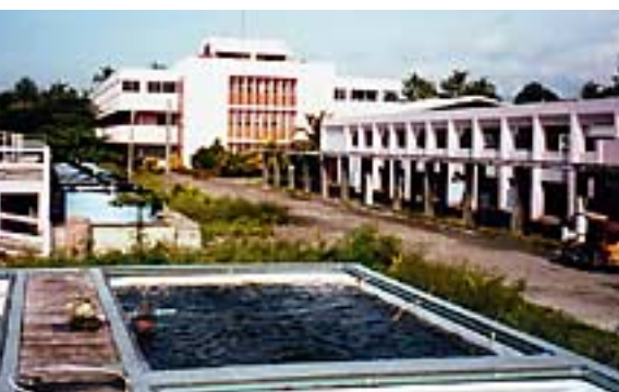
Tigbauan Main Station
