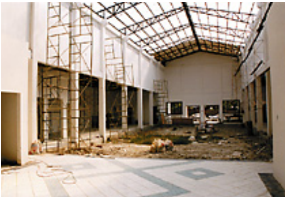
The nearly completed FishWorld (below, right)
