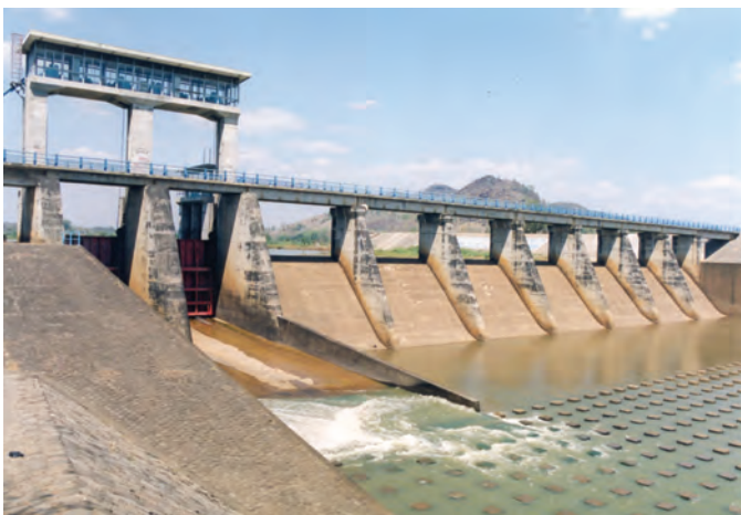
Dam constructed in Solo River
