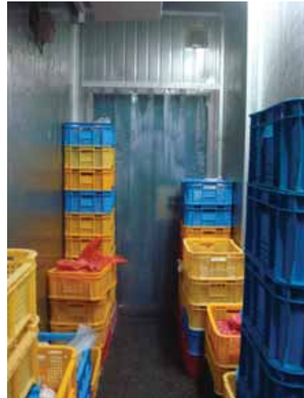
Figure 8 Cooling in air-conditioned room
