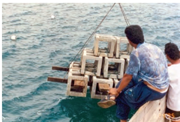
Figure 9. Reinforced concrete ARs installed near Pulau Tioman, Pahang for recreational activities
