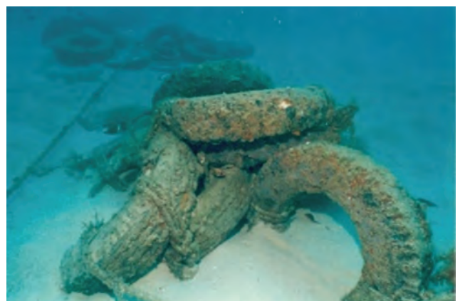
Figure 3. Tire reefs deployed in the open sea of Terengganu in 1990 destroyed by strong water currents (survey in 2007–2008)
