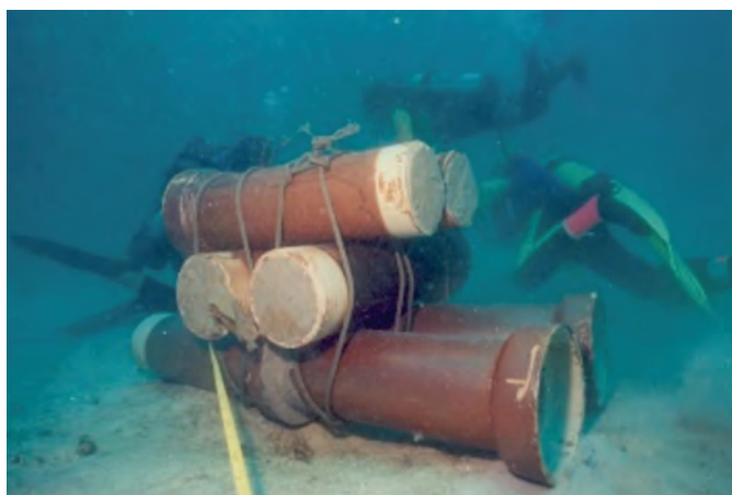
Figure 8. Three-layer ARs using ceramic cylindrical sewerage pipes
