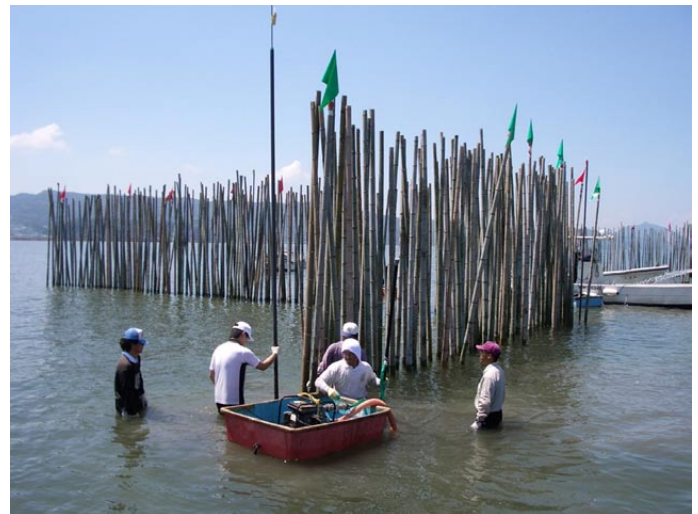
Fig. 4. Bamboo fence installed to promote settlement of drifting larvae (Photo: The Guideline)
