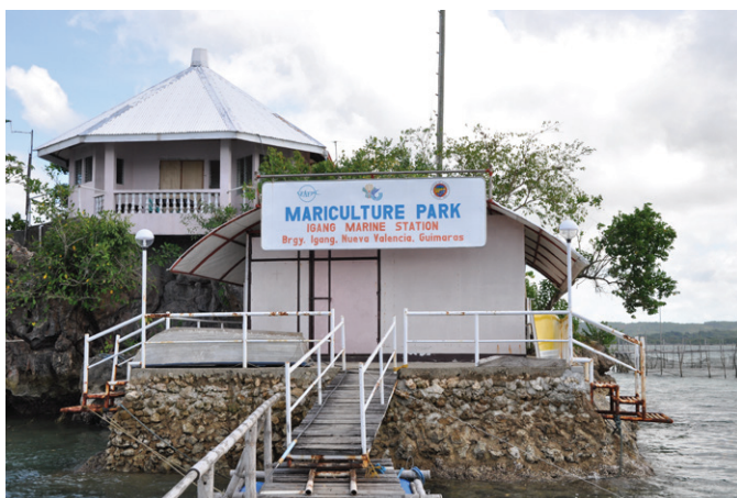
Mariculture Park demonstration and training facility, IMS
