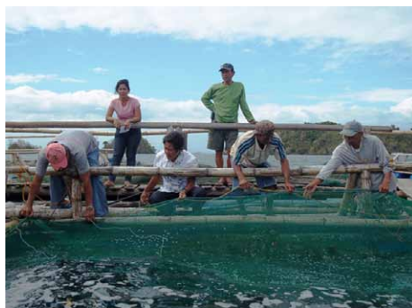
Members of the KAMAMADO install nets for the milkfish cages in Igang Marine Station
