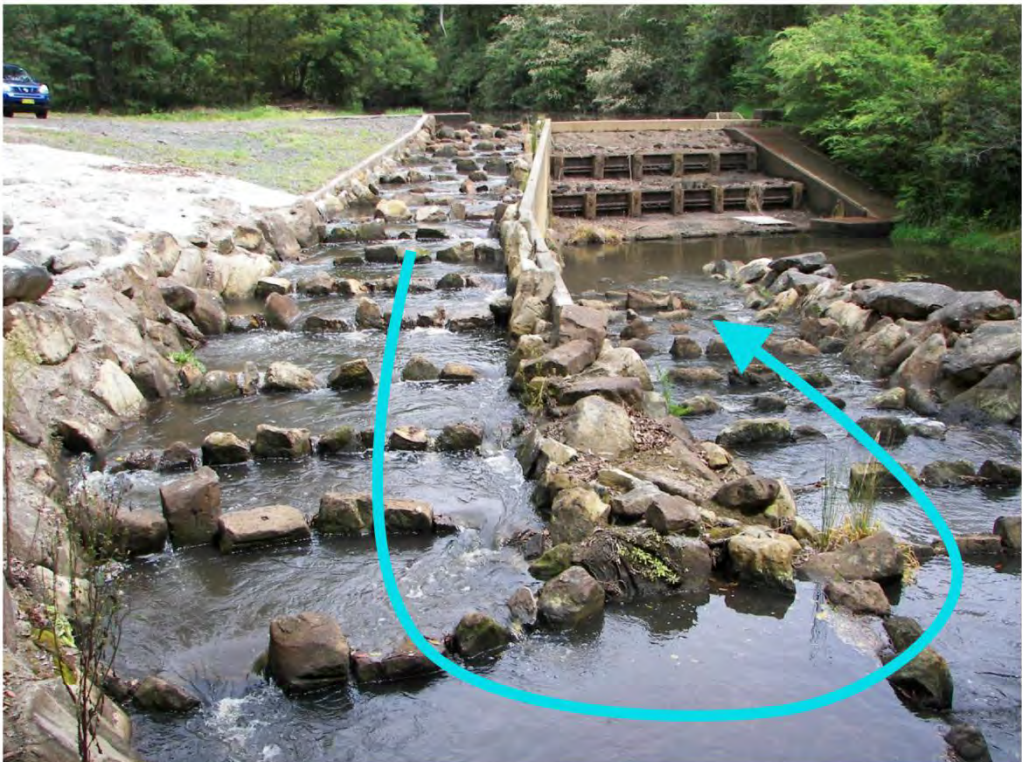
Figure 10. A partial-width rock-ramp fishway with arrow showing direction of flow.
