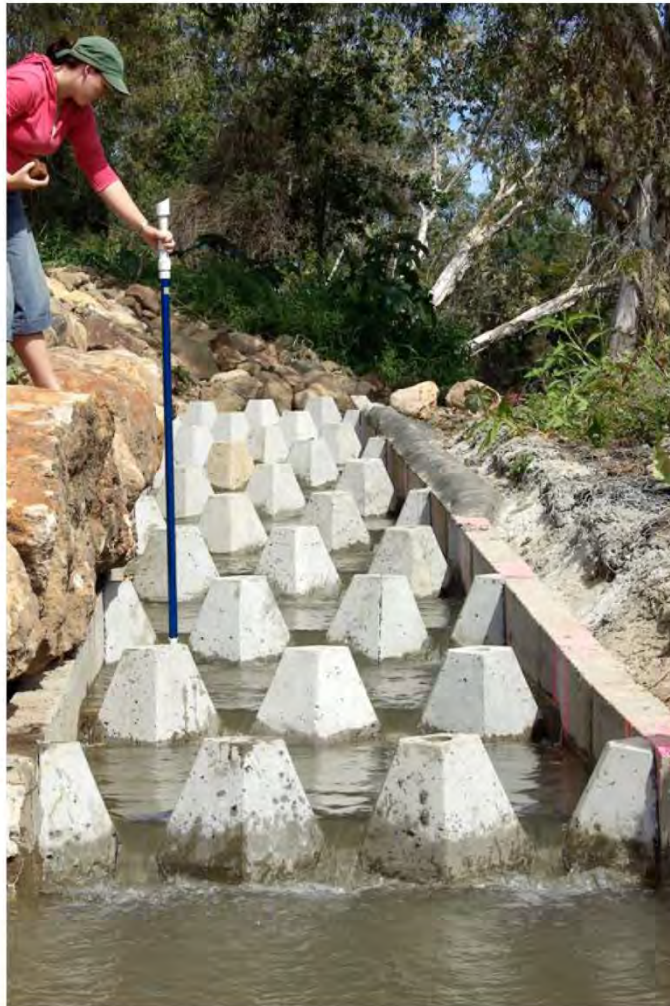
Figure 5. Example of a cone fishway (Photo Courtesy of Tim Marsden).
