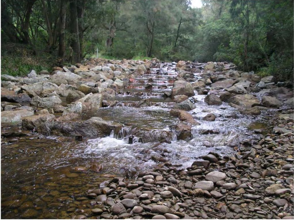
Figure 9. A full-width rock-ramp fishway with central low-flow channel.
