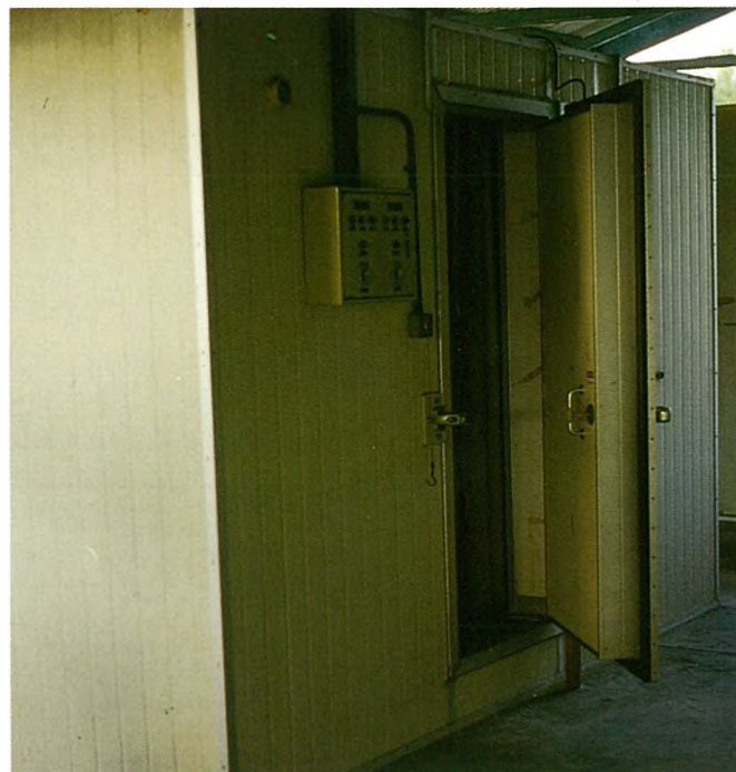
Figure 32. Air blast freezer
