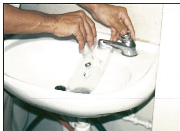
Fig.8 Testing for leaks.
