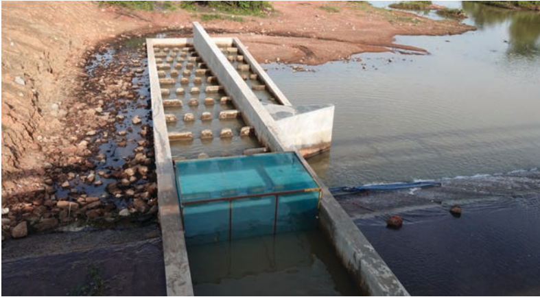
Fish passage in Udonthani Province, Thailand
