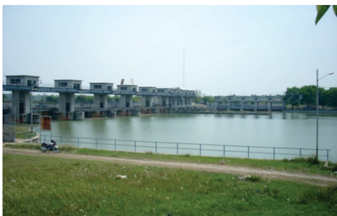
Figure 1. Perjaya Weir, Martapura, Indonesia (Source: BBWS VIII Sumatera Documentation)
