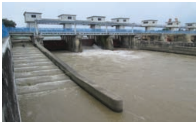
Figure 6. Fish passage in Perjaya Weir, Martapura, Indonesia (Source: Nizar, 2014)
