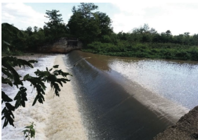
Figure 11. Ea Tul Weir in Srepok River, Dac Lac Province, Viet Nam (above) and the demonstration fish passage being installed (below)
