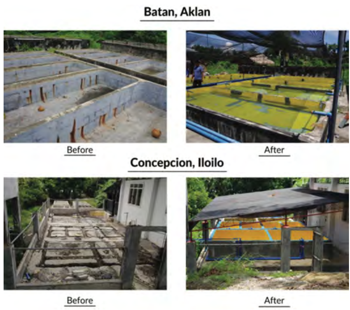
Figure 7. Rehabilitated hatchery tanks in Batan, Aklan; and in Concepcion, Iloilo
