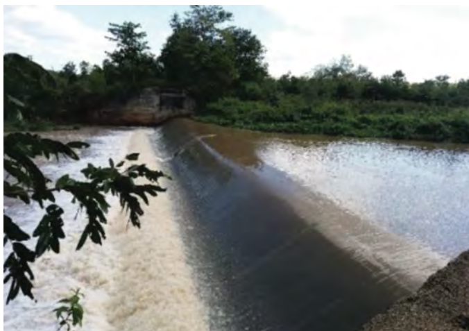
Figure 11. Ea Tul Weir in Srepok River, Dac Lac Province, Viet Nam (above) and the demonstration fish passage being installed (below)
