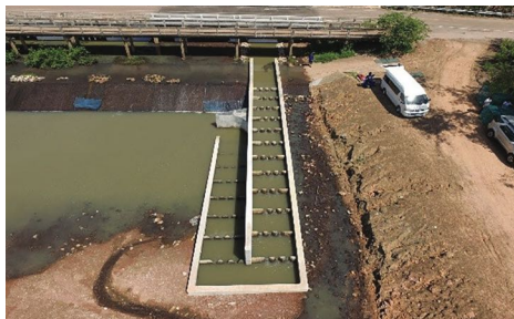
Fish passage construction at Hany Wang Chang Weir, Udon Thani Province, Thailand (left), and setting of fish trap at the exit pool of fish passage to observe its efficiency for fish migration (right)
