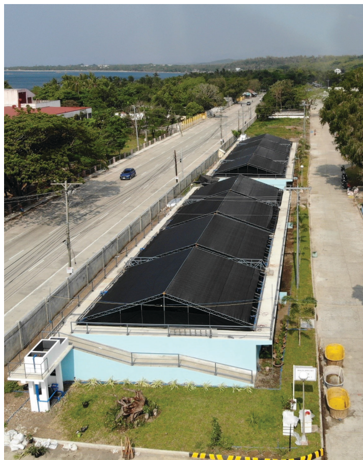
AQD's new broodstock tank facilities at its Tigbauan Main Station
