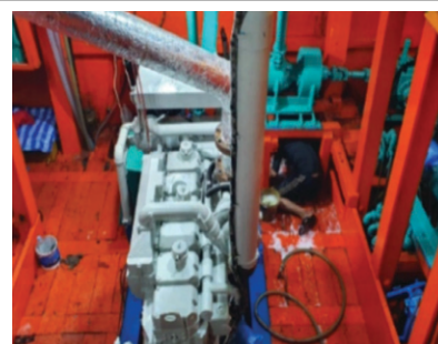
Engine installation in the engine room
