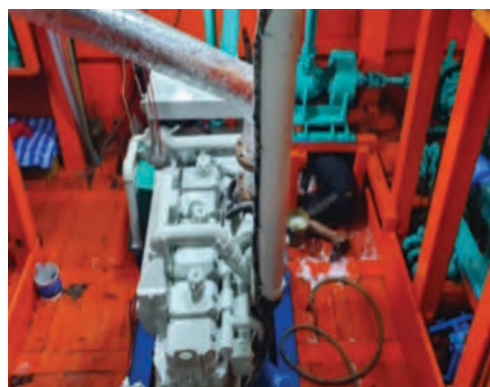
Figure 3. Installation of engine in the engine room
