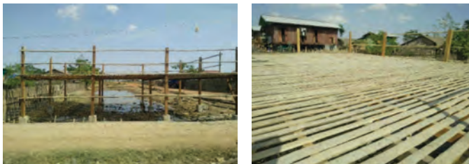
Figure 7. Fish drying rack constructed in Aung Kan Thar Village with support from SEAFDEC
