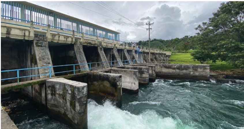
Lake Ranau Regulating Dam
