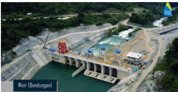
Perjaya Weir, Martapura, South Sumatra (above) and Sulawena Weir, Poso, Central Sulawesi (below) in Indonesia
