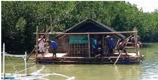
Newly-built floating hut serving as guarding and sampling post
