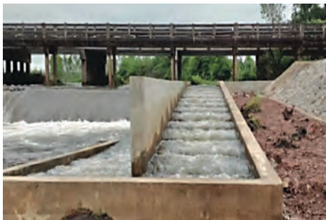
Fishway in Hany Wang Chang Weir constructed at in Sangkom Sub-district, Thailand
