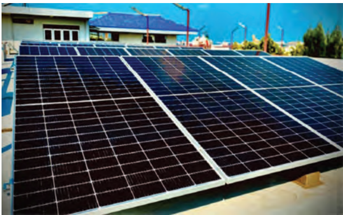
Figure 2. Solar panels installed on the rooftop of one of the SEAFDEC/TD office buildings in 2022
