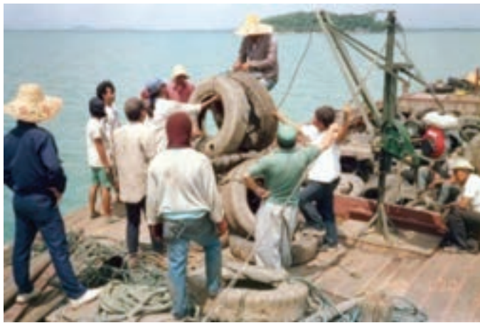
Figure 1. Tetrahedral tire reefs developed in Malaysia in 1975
