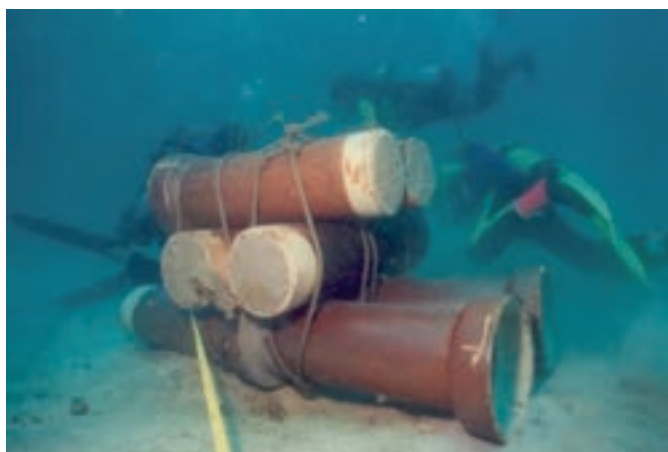
Figure 8. Three-layer ARs using ceramic cylindrical sewerage pipes
