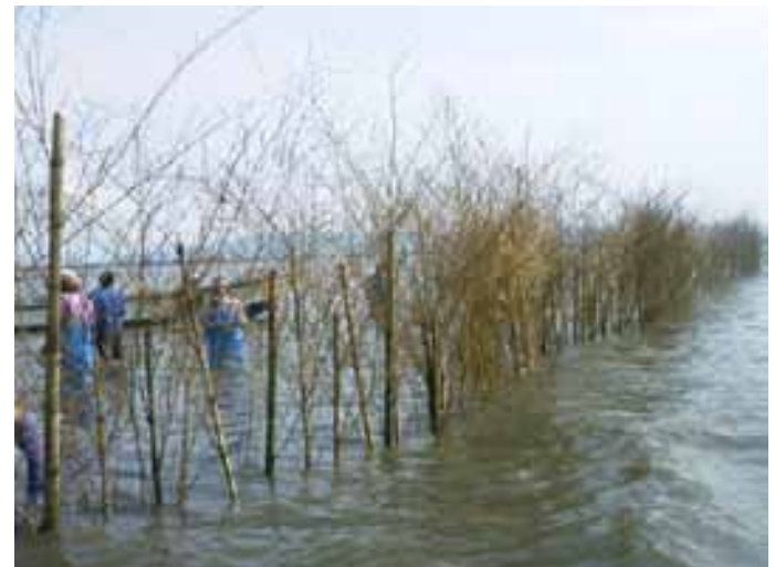
Fig. 10a. Bamboo fence installed to promote settlement of drifting larva (Source: Kumamoto City and Matsuo Fishery Cooperative)
