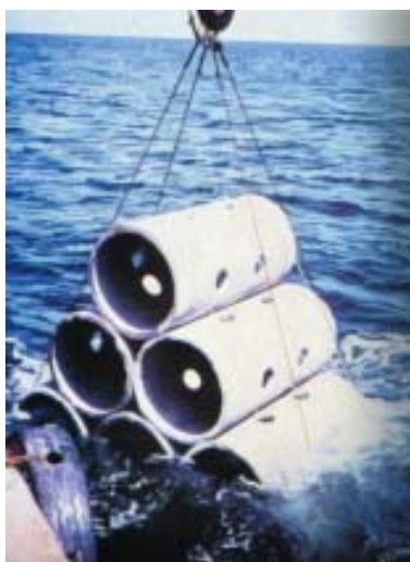
Installation of perforated concrete pipes as ARs
