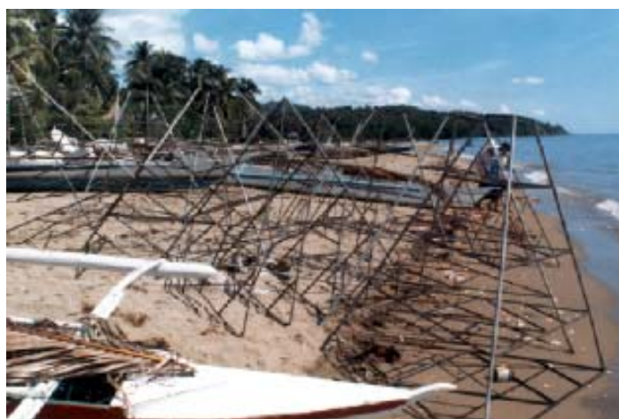
Galvanized iron pipes soldered into pyramid shape to be deployed as AR, stored on the beach, at Carmen, Philippines
