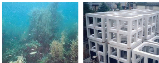
Examples of AR structures in Japan: Left: to create seaweed beds; Right: to promote coastal fisheries (Source: Sato, 2009)
