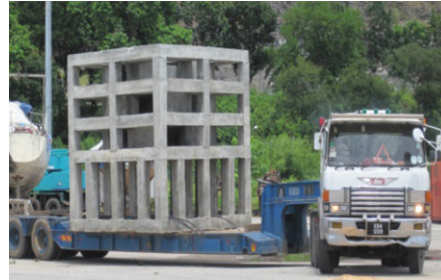
Fig. 2. Soft-bottom juvenile enhancement AR (size: 3.75m x 3.75m x 3.85m; weight: 32 MT)
