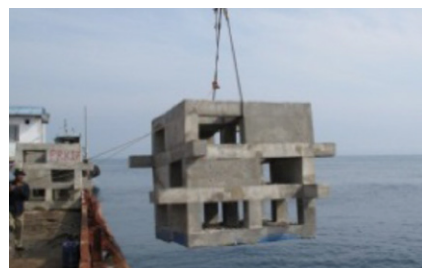
Fig. 5. Installing a cube anti-trawler AR by DoFM
