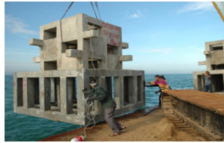
Fig. 1. Soft-bottom anti-trawler AR (size: 3.75m x 3.75m x 3.85m; weight: 32 MT)
