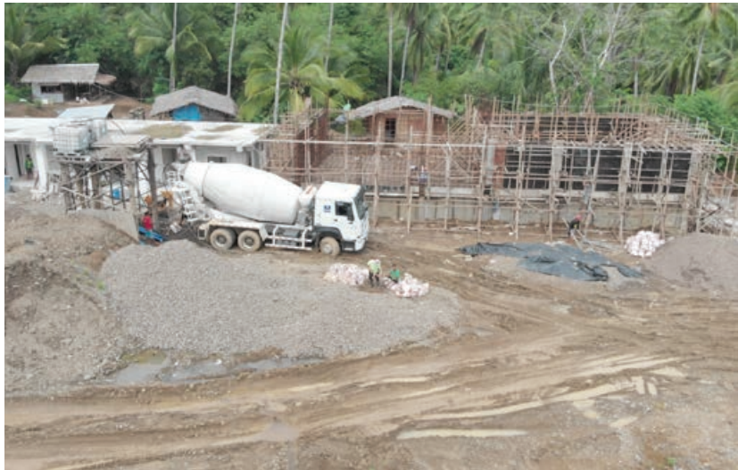
On-going construction of the multi-species hatchery in Lingig, Surigao del Sur
