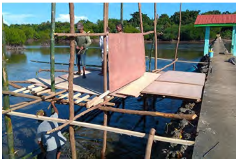
On-going construction of abalone hatchery on stilts alongside the foot walk connecting Molocaboc Dacu and Diut, Sagay Marine Reserve, Negros Occidental, Philippines
