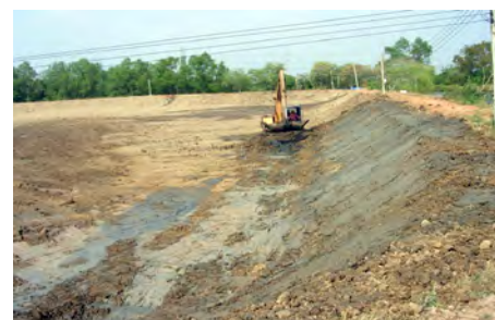
Figure 17. Packing dikes properly to prevent pond water from leaking
