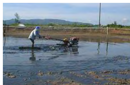
Figure 16. Dredging pond bottom to remove waste materials
