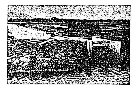
A sluice gate should be located near the water source in order to take in water during high tide. Another sluice gate is located at the opposite end of the pond. The gates should be about 1 to 2 cm. thick. The number of gates depends on the size of the pond, i.e., two gates for a 4 ha pond and three to four gates for an 8 ha pond. The gates should be watertight and have a strong foundation in the form of a cement base.
