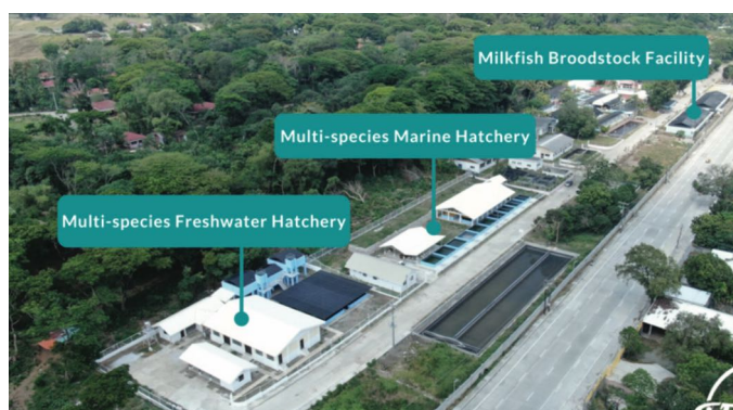
Figure 10. The newly completed hatchery systems at SEAFDEC/AQD Tigbauan Main Station, Iloilo, Philippines
