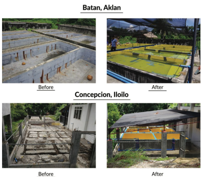
Figure 7. Rehabilitated hatchery tanks in Batan, Aklan; and in Concepcion, Iloilo
