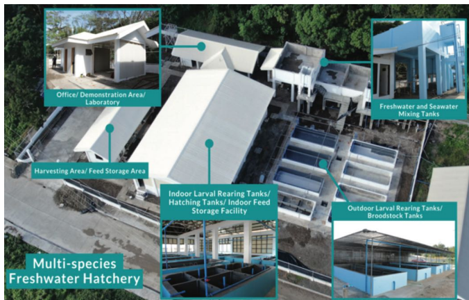
Figure 9. The newly constructed freshwater multispecies hatchery at SEAFDEC/AQD Tigbauan Main Station, Iloilo, Philippines
