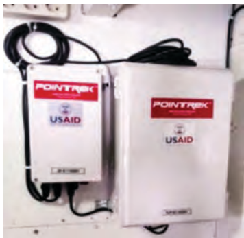
Figure 14. Pointrek/ Inmarsat Two-Way Communication Vessel Monitoring System (VMS)
