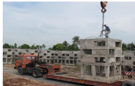
Fig. 3. Soft-bottom cuboid AR (size: 3.0 m x 3.0 m x 3.85 m; weight: 22 MT)
