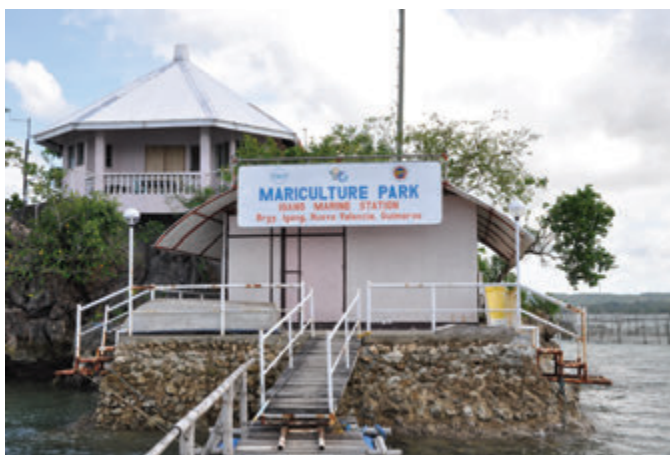
Mariculture Park demonstration and training facility, IMS
